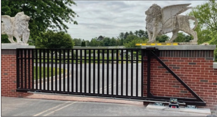
Diagonal trussing in the vertical dimension is needed for all gates. A simple diagonal in the tail section will work for many “smaller” gates.
