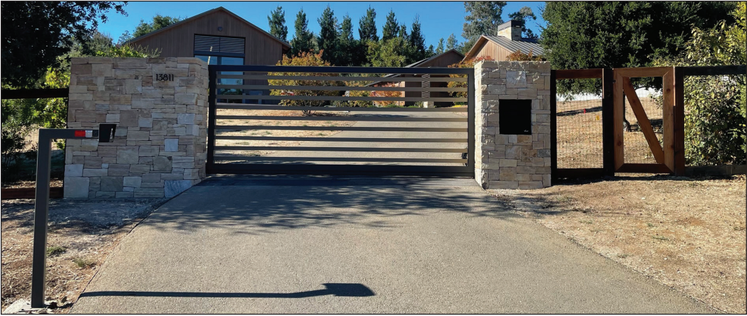
This sleek, lightweight sliding gate at a residence in California used the Duragates CGS-250.8M model. The homeowner wanted it automated so they chose a FAAC gate operator. The keypad out front allows for easy entry to the property. The tail end of the gate is nicely hidden behind a stone wall hiding the gate hardware from the street.
