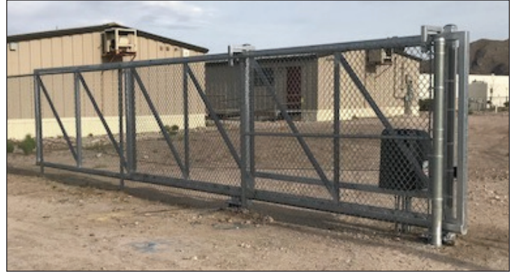
Diagonal bracing in each section should be used for large gates with a 30 ft or greater opening.
