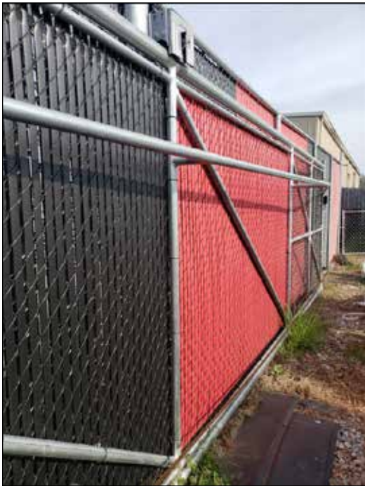
Diagonal trussing in the vertical dimension is needed for all gates. A simple diagonal in the tail section will work for many “smaller” gates.
