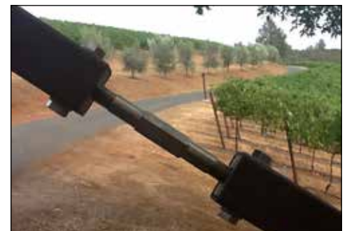
The top corner of the gate will rise and fall as tension is adjusted on the tension bar.
