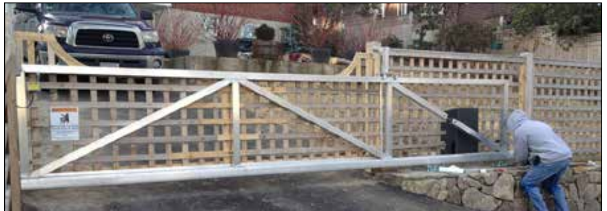
Example of a wooden gate with aluminum frame, well trussed and supported.
